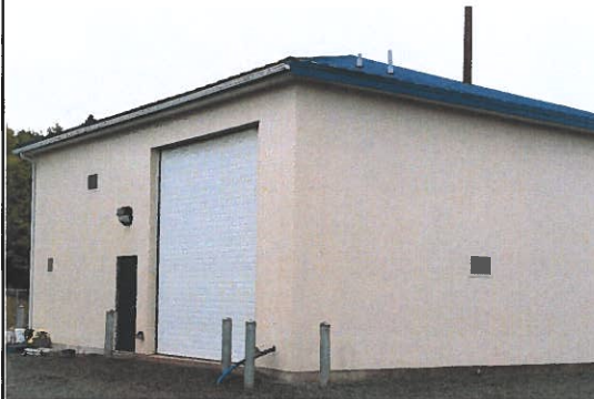
Water treatment plant. Photos: Peter Cottingham
