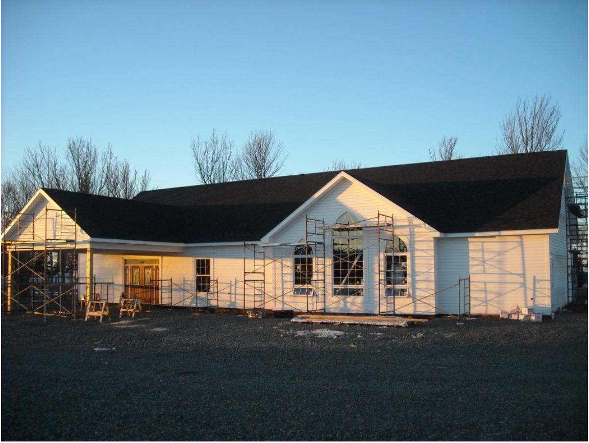
Church under construction.
